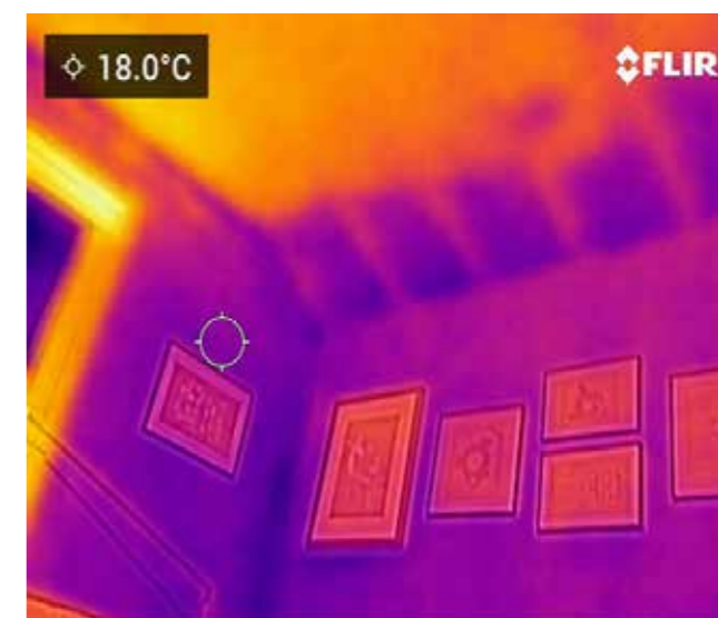
An infrared thermographic image showing loft insulation that has not been extended to the edge of the roof, letting heat escape
