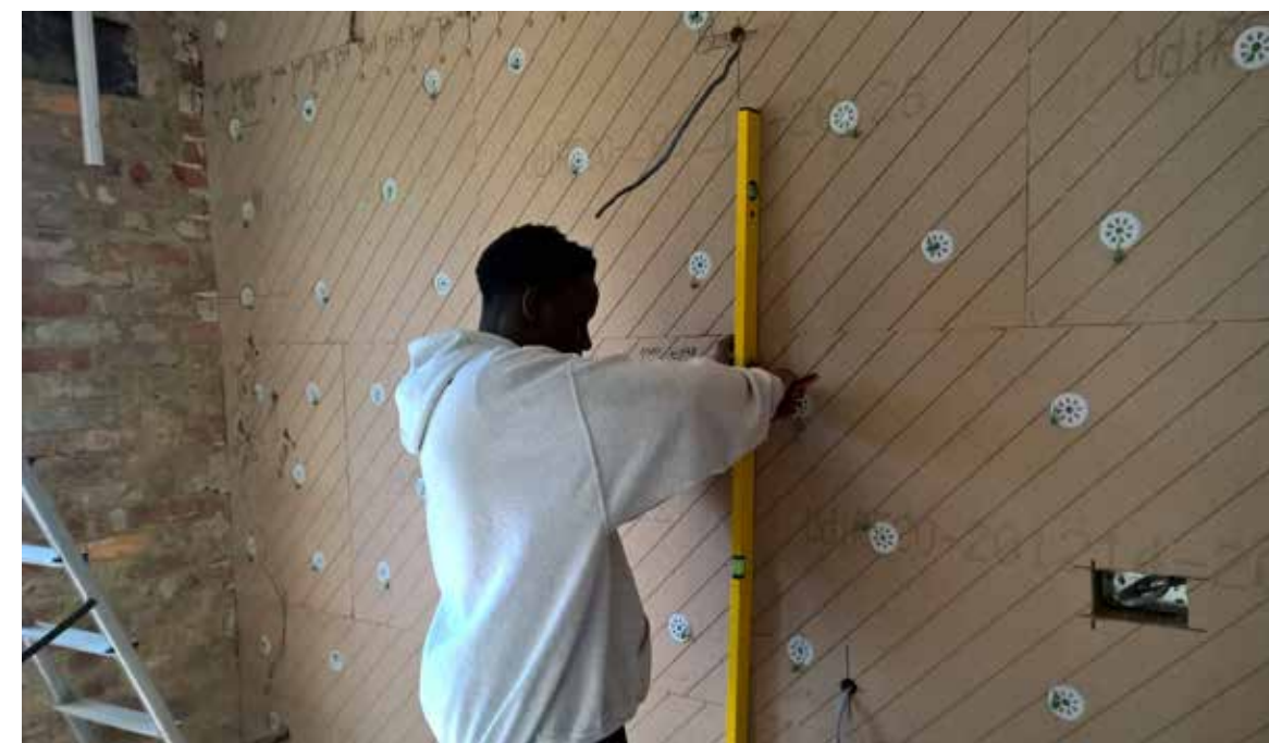
Installation of wood fibre insulation boards internally (Source: Back to Earth & ASBP)
