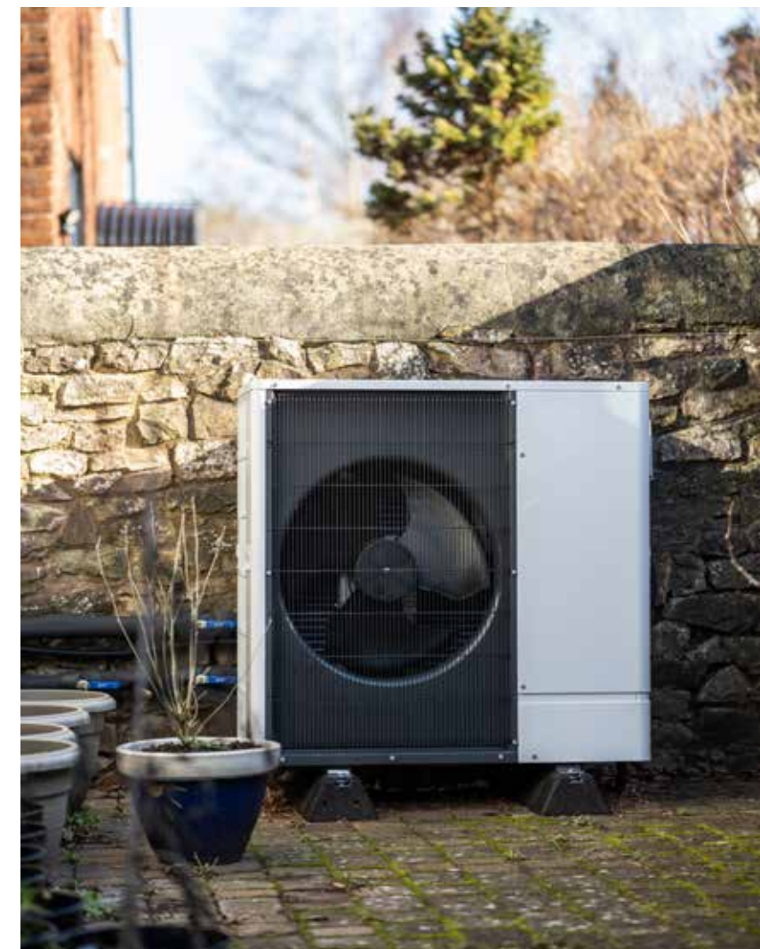
Image of an external condensing unit for an ASHP. Source: Rob Coombe
